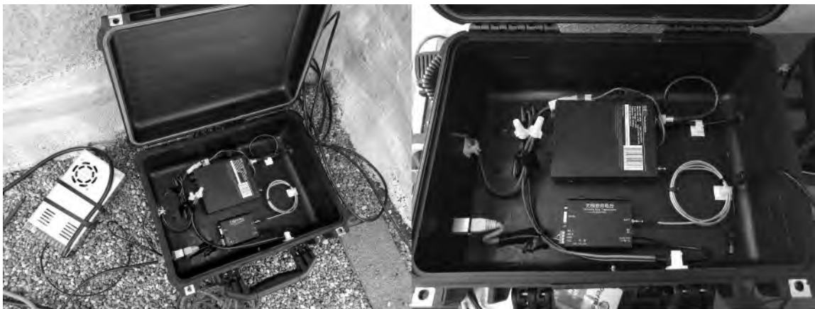
Figure 3: High power base station transmitter setup. While RS-485 communications were performed with the Category 5e cable, power had to be supplied by a nearby 12V power supply (silver metal box on left) due to the power demands of the 25W amplifier.
